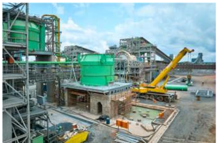
The installation of the scavenger-cleaner flotation cell at the Phase 2 Concentrator is nearing completion. The de-bottlenecking program is expected to be complete in Q2 2023.
