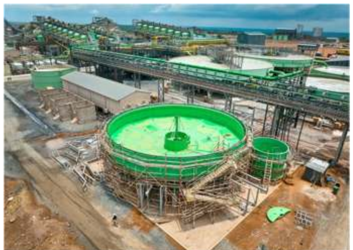
The installation of the scavenger-cleaner flotation cell at the Phase 2 Concentrator is nearing completion. The de-bottlenecking program is expected to be complete in Q2 2023.
