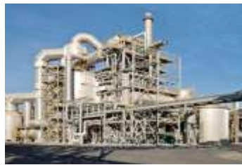
Fig.3: Ma'aden Aluminium Refinery
